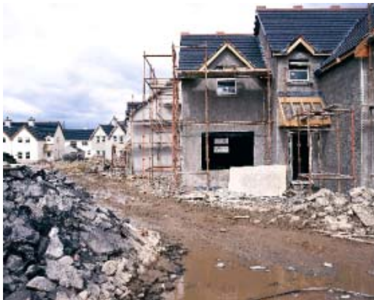
Photograph 1 New housing construction
