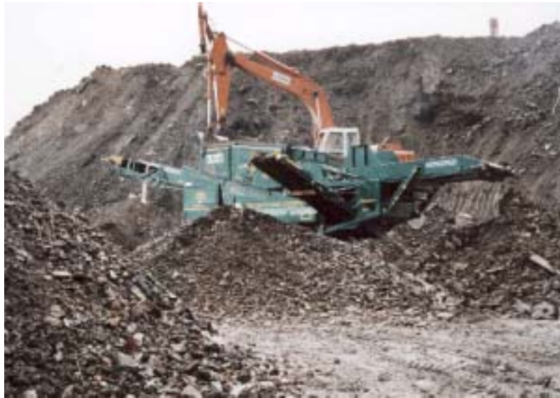
Photograph 2 Construction and demolition waste recycling at Ballealy Landfill
